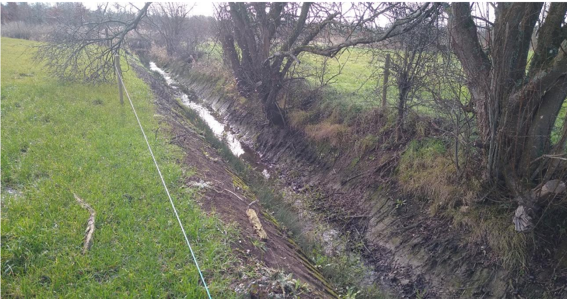
Figure 4-5: Drainage ditch (FW4) to the west of the site. Note the presence standing water backfilling from the river
